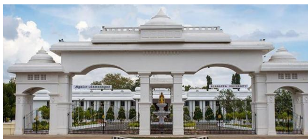
University Administrative Building
